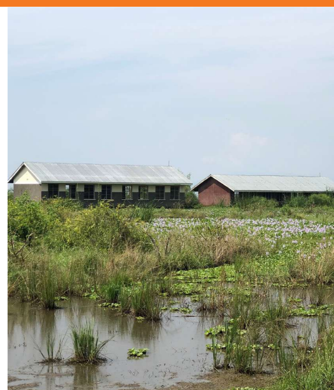
Two classroom blocks of Wanseko Primary school Annex inundated by flood water from rising water levels of Lake Albert.
