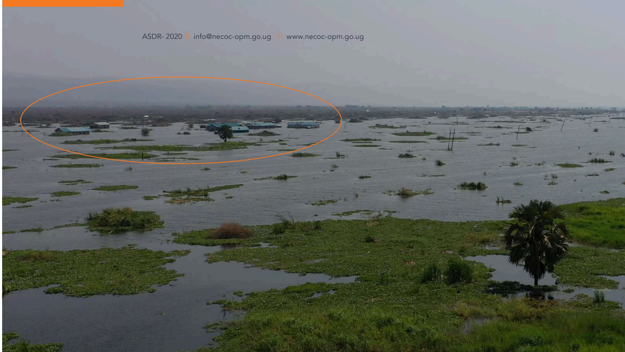
Newly rehabilitated Butiaba Health Centre III in Buliisa District submerged by floods resulting from rising water levels of L. Albert. Notably, it is important for all stakeholders to undertake risk assessments for any development or social service project.
